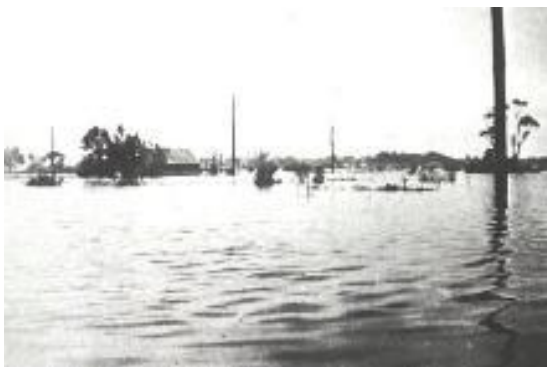
Figure 2: Early photo of flooding at Narrabeen Lagoon
